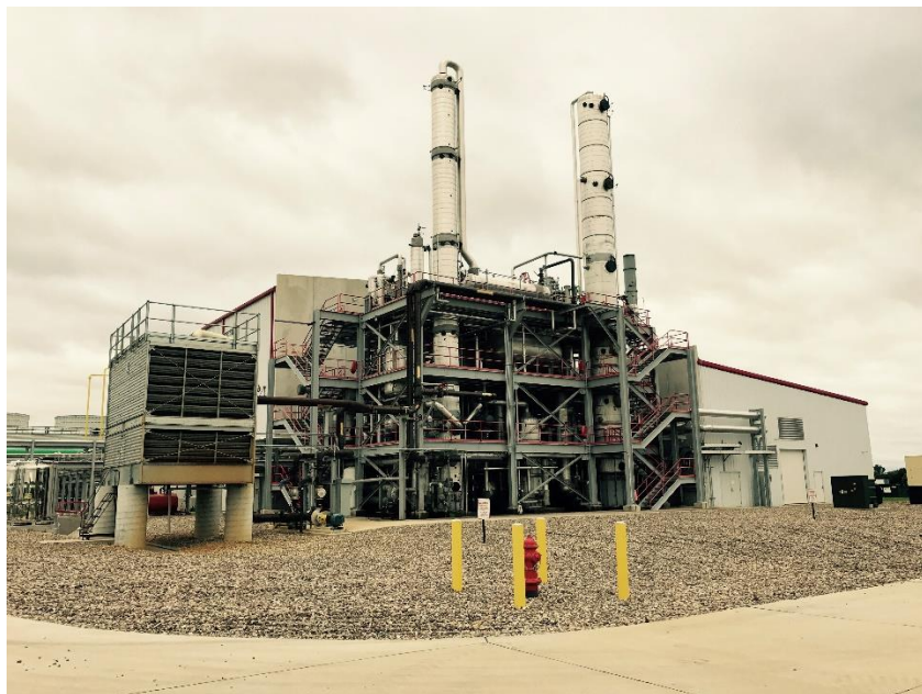
CHS, Inc. Super Biodiesel plant co-located with 110mmgy Ethanol plant, Annawan, IL
